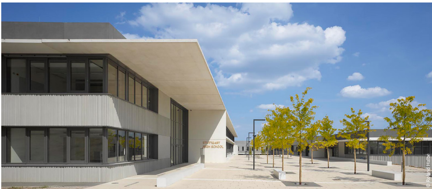
American High School & Elementary School, Stuttgart-Böblingen
